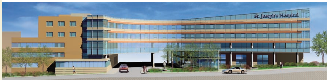
The new patient tower at St. Joseph's Hospital.
